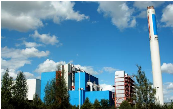
Image FA2212-01: Incinerator plant, Weisweiler GmbH & Co. KG
