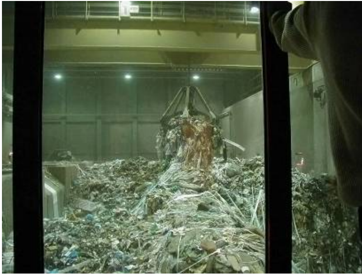
Image FA2212-06: Incinerator plant, Weisweiler GmbH & Co. KG
