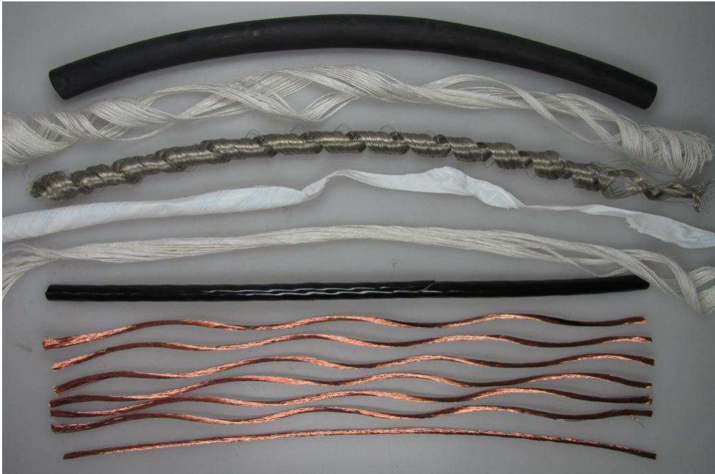
Overview of the dissected pieces of the cable no.1.2, point of the middle point after 17.099.049 cycles.
