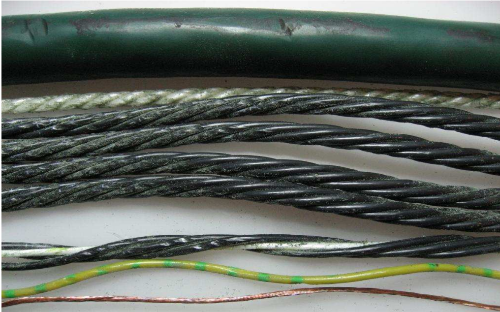
Overview of the dissected pieces of cable of no. 1.1 CF5.10.25 after 41.538.456 strokes
